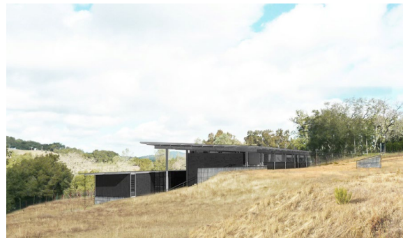
The height of building steps down with the landscape, mimicking the staggered slope of the site.
