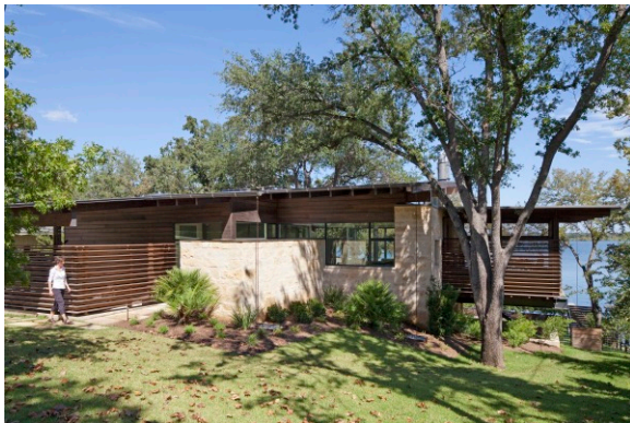
A series of built and landscape elements work together to ground the building to the hillside. The layered effect also creates visual interest by assigning levels of hierarchy to the overall building composition.
